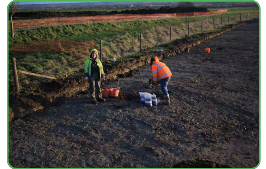
Indie and Danny excavating pits in Area C
