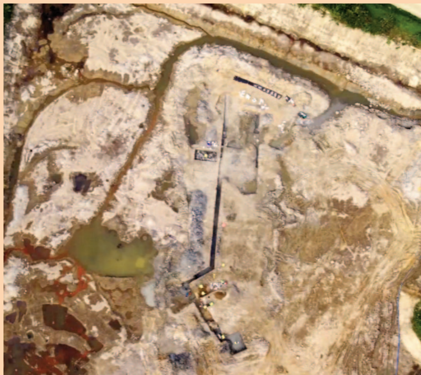
Right: Drone view of site during excavation
