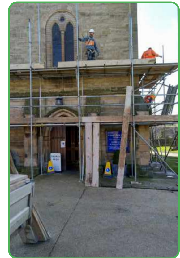
With the arrival of Covid-19 in the UK and the national lockdown in March 2020, the delivery phase was postponed, but restoration work at the church continued...
