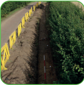
Plate 17.1 - Mid-excavation facing E, showing aspect of trench adjacent to main driveway.
