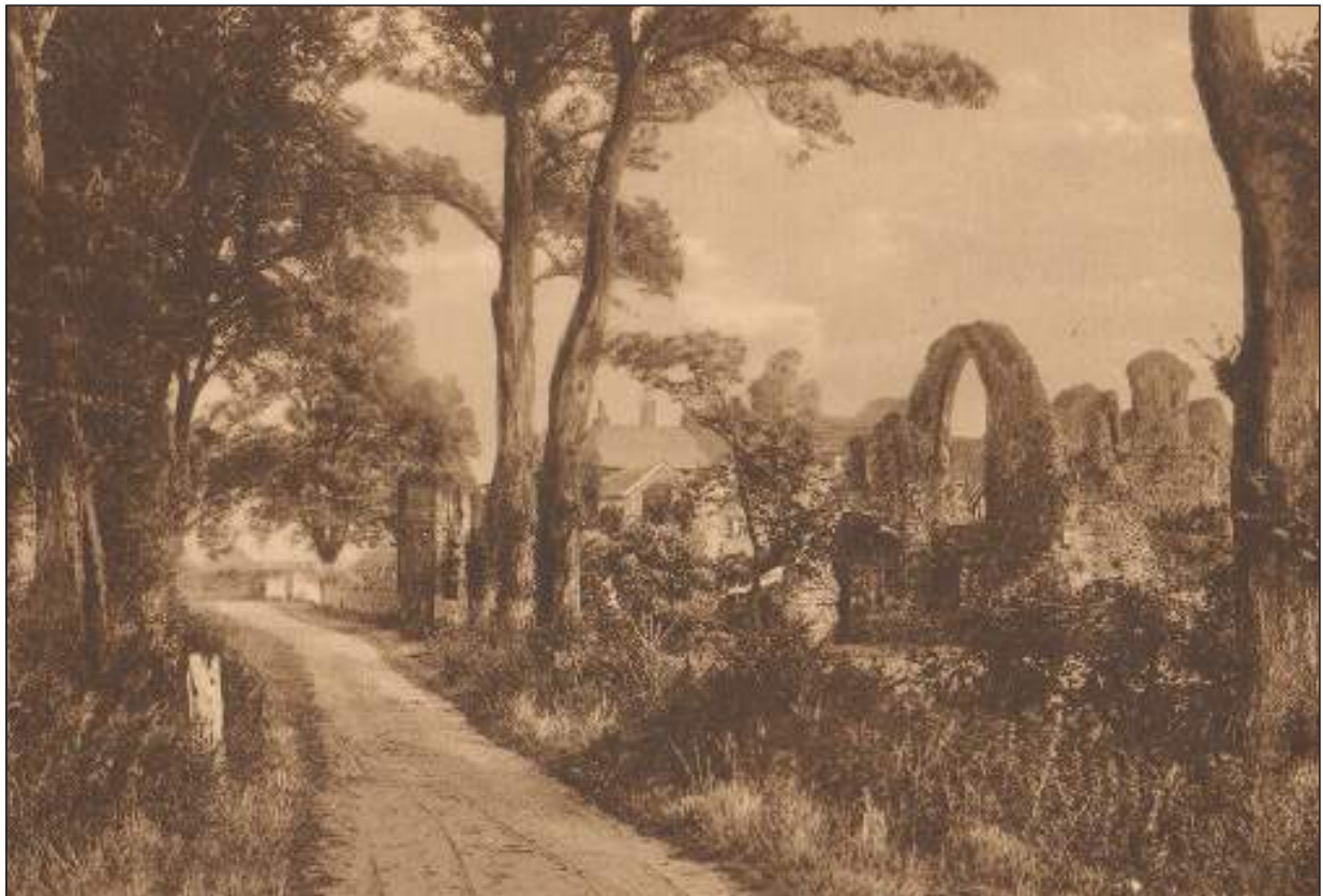
Plate 19.3 – Postcard from c.1900, illustrating vegetation adjacent to the southern site entrance, and likely truncating the medieval wall observed in Trench 20
