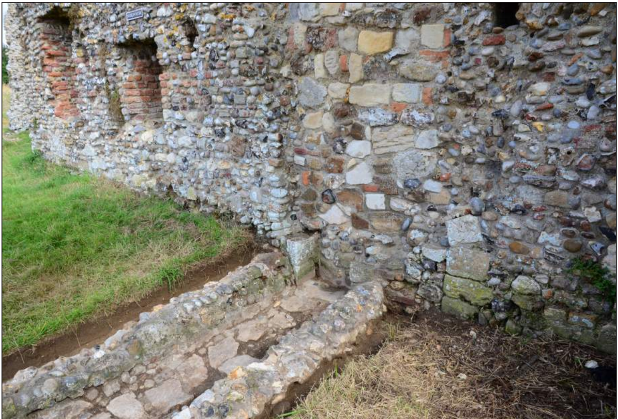
Plate 17.2 - Reconstructed Reredorter drain showing association with original monastic wall, post-excavation, facing NW
