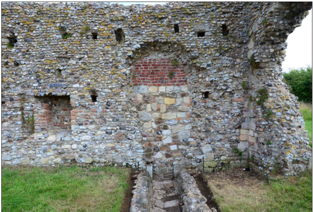
Plate 17.4 - Showing relationship of drain to filled-in arch in Reredorter wall, post-excavation, facing N
