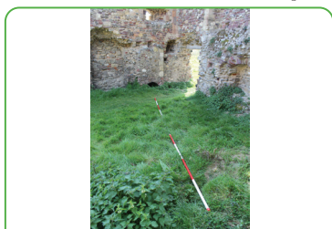
Plate 1.4 The Undercroft, indicating the passage of the drain, facing south-west
