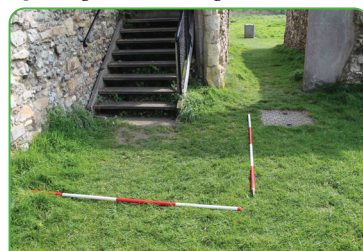
Plate 1.5 Cloister, base of day stair and inner wall, facing south
